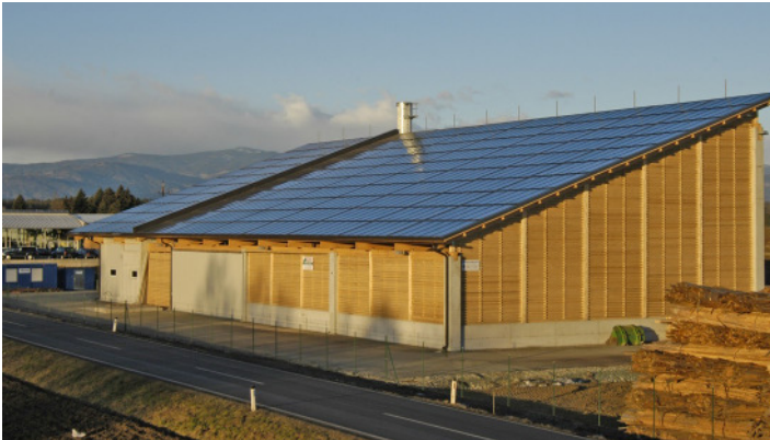
Photo: LEV Gleinstätten District heating
